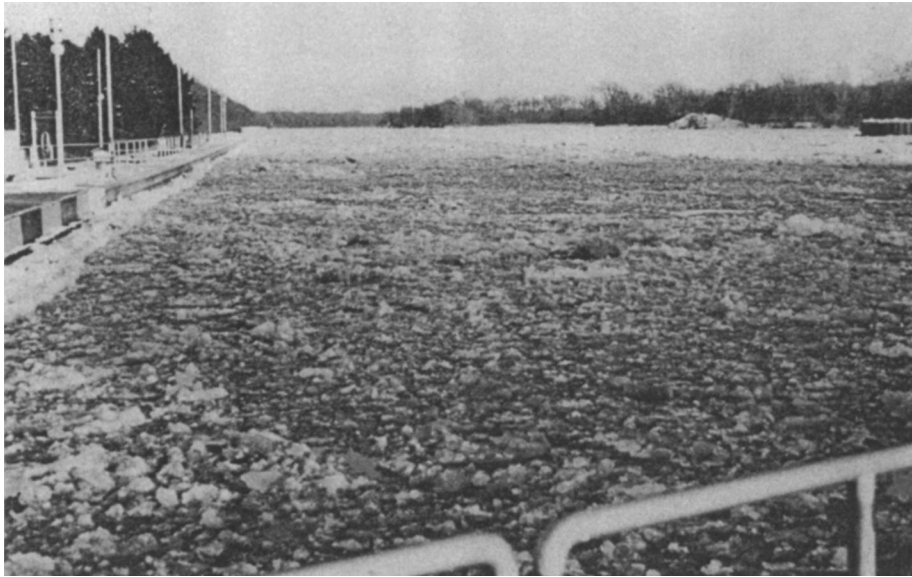
Figure 3-2. Ice accumulation in the upper lock approach area.
