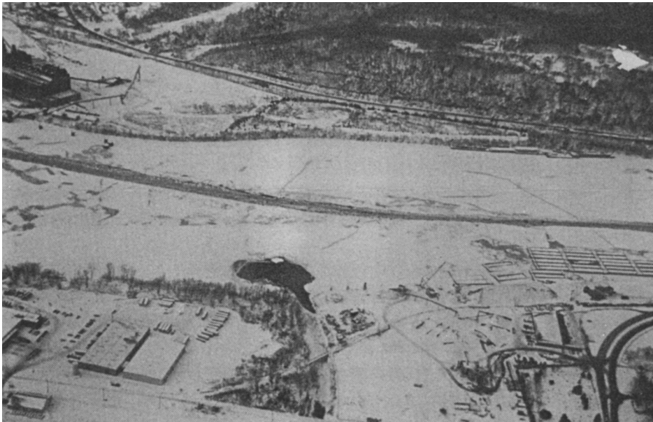
Figure 3-14. Navigation track in the middle of the channel, with a fleeting area at the near bank. Traffic using the fleeting area can breakfree large floes that can move out to block the track.
