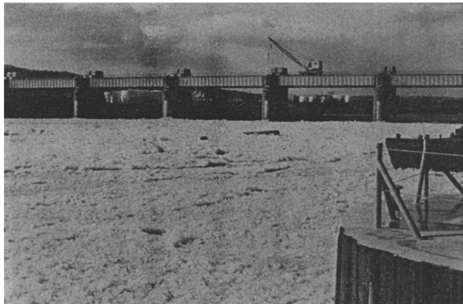
Figure 3-6. Ice accumulation upstream of the gates of a navigation dam.
